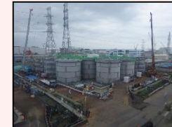
Start of dismantling in H1 east area
