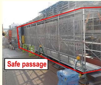
Installation of roofed safe passage
