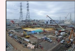
After dismantling in H1 east area
