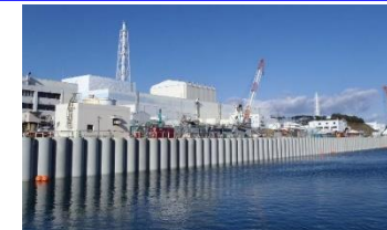
(Sea-side impermeable wall)
