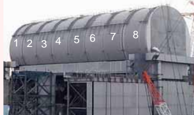
Installation of dome roof (February 21)
