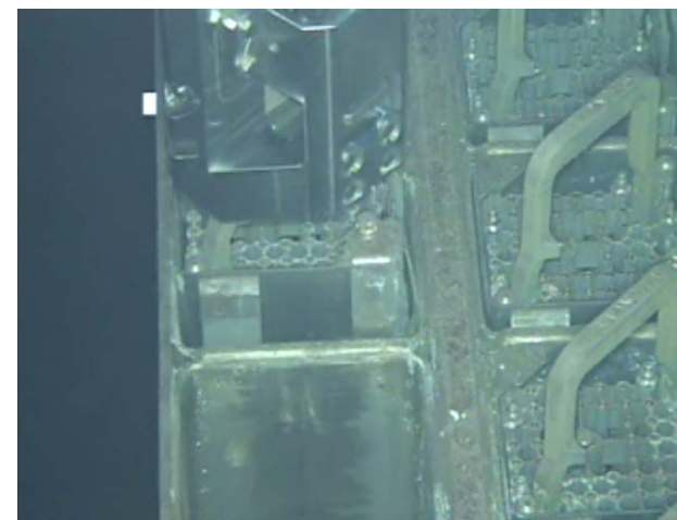
Fuel removal operation (Nov. 18)
