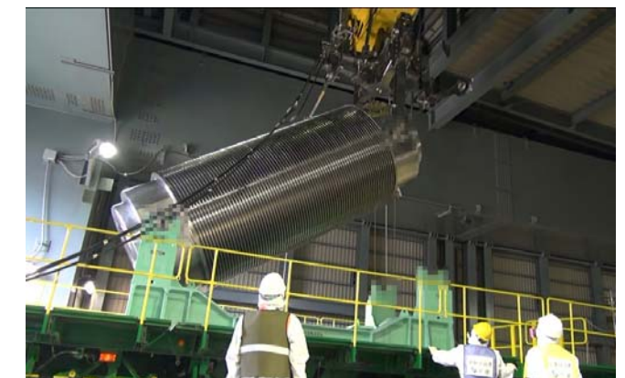
Loading of on-site transfer container on the trailer (Nov. 21)
