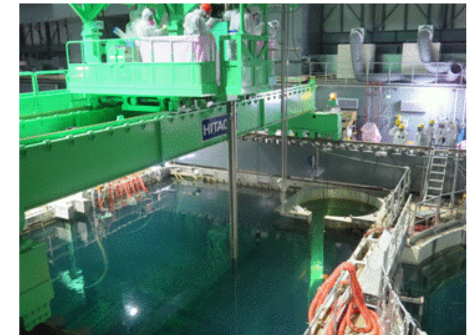
Operation of fuel removal (Nov. 18)
