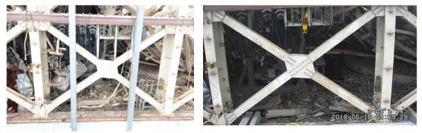
Removal of surrounding steel trusses (left: before removal, right: after removal)
