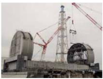
Unit 3 Fuel removal cover (dome roof) installation (September 6)
