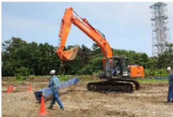
Debris removal / Road restoration training (Debris removal)
