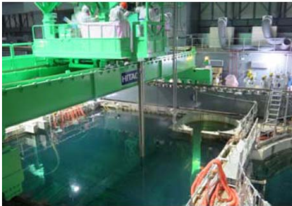
Fuel removal from spent fuel pool
