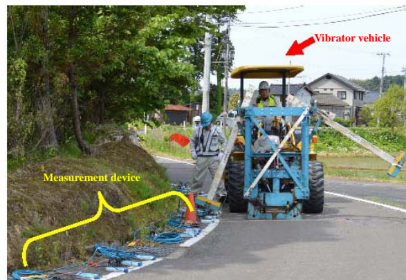
Subsurface prospecting in the vicinity of the plant site (Itsukaichi District)
