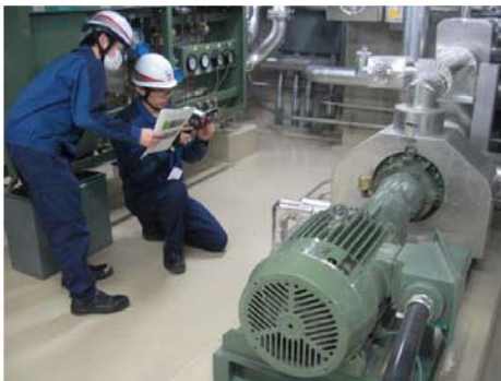
Data collection administered by operators (Example: Diagnosis using infrared thermograph)
