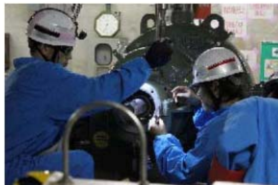
Cooling Water Pump Restoration training (bearing assembly)
