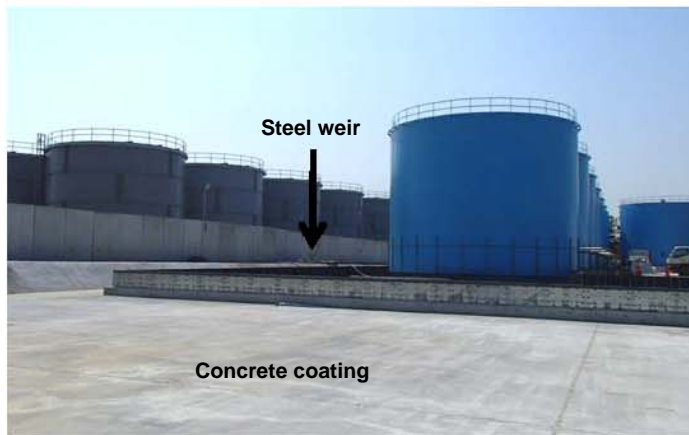
Work progress for double structure tank weirs and coating inside weirs
