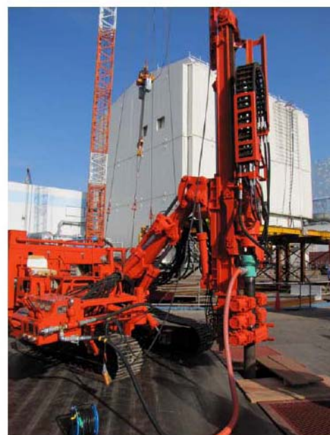
Status of chiller piping installation work
