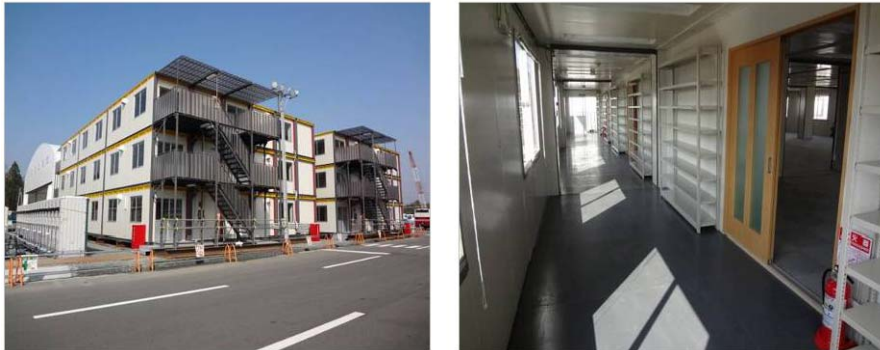
Temporary ex-site rest station (External view / Inside)
