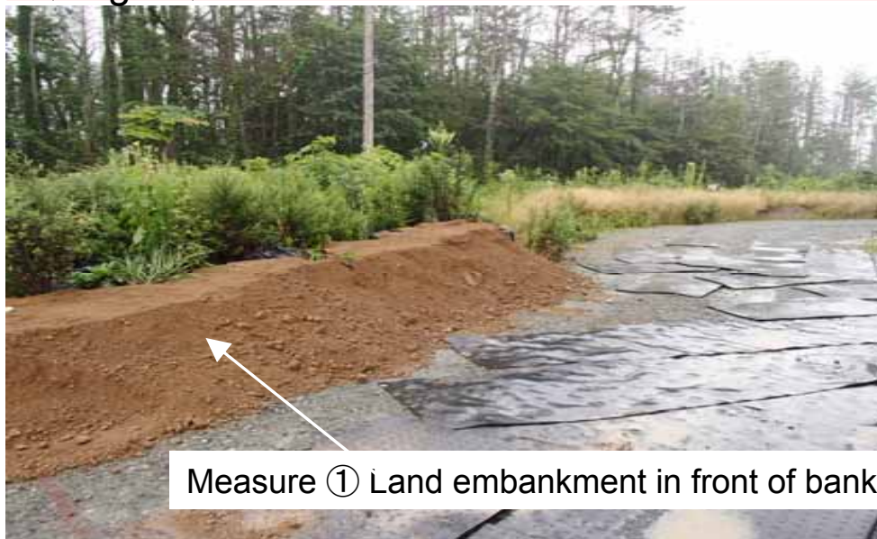
Measure ③ Setting up waterproof sheets
