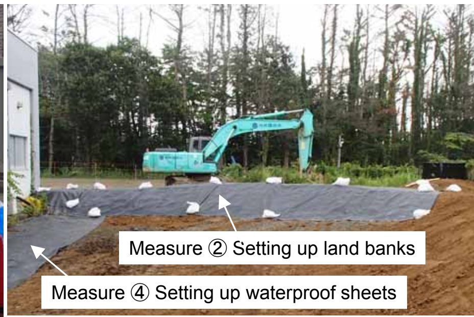
Measure ③ Setting up waterproof sheets
