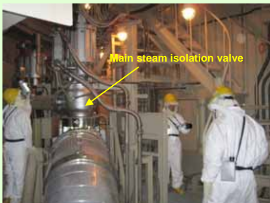
7. Visual inspection (Photo taken on May 10, 2012)
