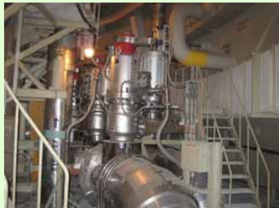
2. Inside PCV (Main steam isolation valve) (Photo taken on April 17, 2012)
