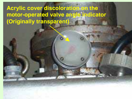
12. Acrylic cover discoloration on the motor-operated valve angle indicator (Photo taken on March 13, 2012)
