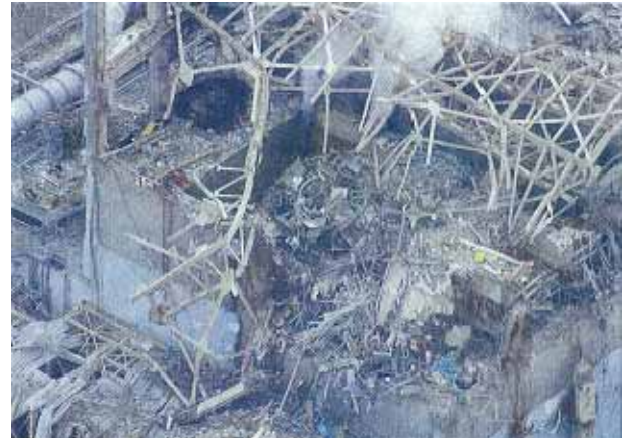
Figure-2.3 Situation of Northwest Floor Slab on 5th Floor
