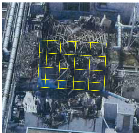
Figure 4-1 Damage Conditions of the Reactor Building of Unit 3 (Elevation)
