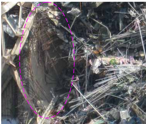
West Side Wall of Dryer Separator Pit
