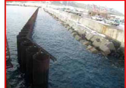
steel sheet pile ( Image )
