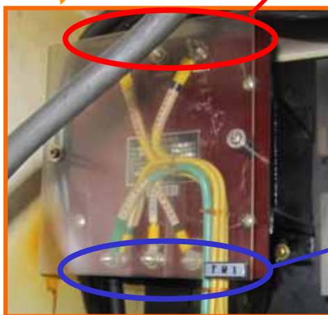
Auxiliary transformer for IA dryer control circuit
