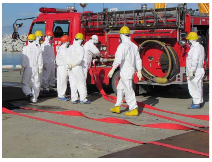
Water injection to the reactor by using pump of fire truck (at around Shallow Draft Quay) (3)
