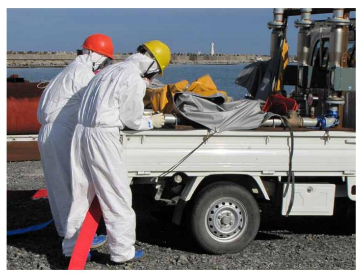
Water injection to the reactor by using pump of fire truck (at around Shallow Draft Quay) (4)
