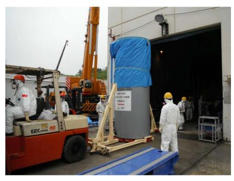
2nd Cesium adsorption apparatus (carrying vessel into building)
