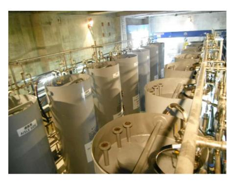
2nd Cesium adsorption apparatus No1
