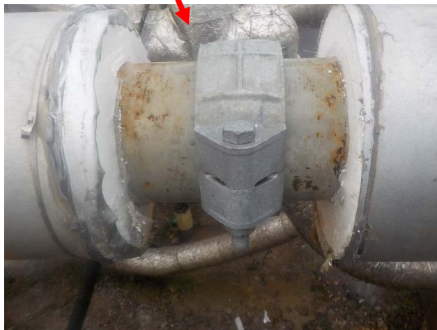
Source of the leakage identified on December 20 (one of the header pipe joints)
