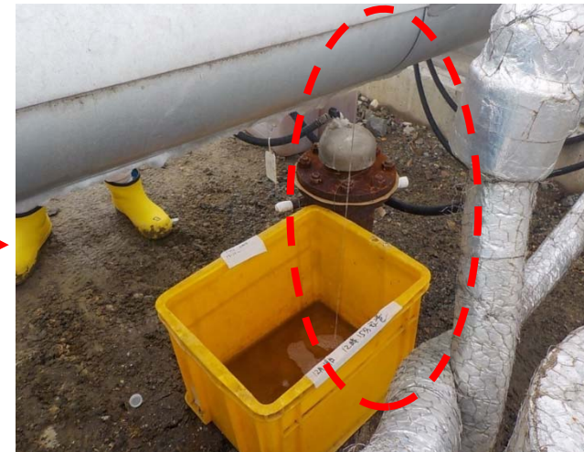
Coolant leakage on December 19 (a joint of covering material near the source of the leakage)
