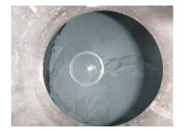
←Inside Absorption tower 4B (image taken from the inspection chamber at the upper part) Gray colored sediment was confirmed on the surface of Absorbent 2 (estimated to be carbonate).
