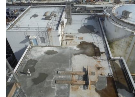
Roof of the Unit 3/4 additional service building
