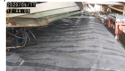
After filling with air mortar (June 11)
