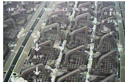
Fuel and upper portion of the fuel rack
