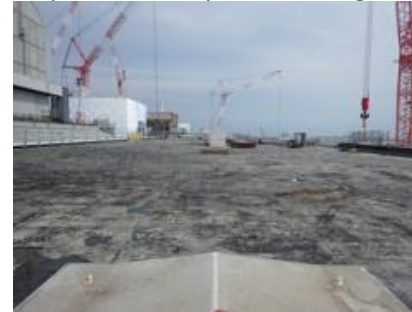
Rooftop of the Unit 3 turbine building
