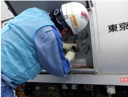
Cable connection inspection (power supply truck operation training)
