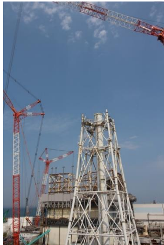
Exhaust stack after dismantling (May 2020)
