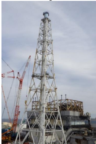
Exhaust stack prior to dismantling (July 2019)
