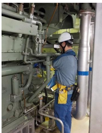
Changing lubricating oil tank refueling procedures to reduce the risk of oil leaks (Kashiwazaki-Kariwa) Right: Opening tank refueling valves Left: Checking tank refueling levels
