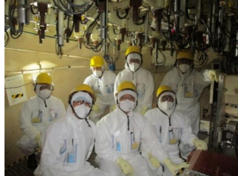
At the bottom of the Unit 5 reactor pressure vessel
