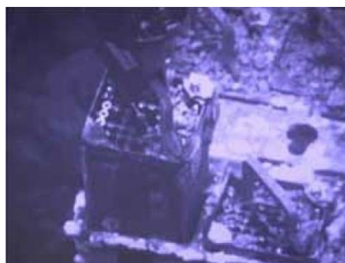
Fuel removal work
