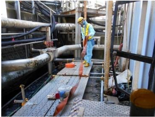
Laying hoses (training on responding to reactor coolant injection equipment damage)
