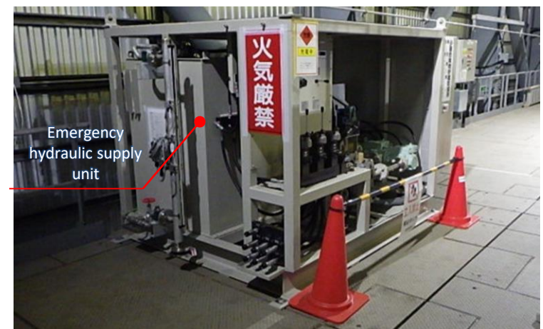
Emergency hydraulic supply unit on August 5, 2025
