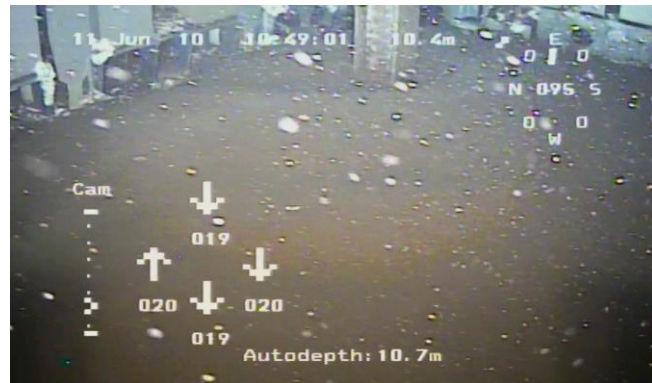
Sandy deposits at the bottom of the cask pit
