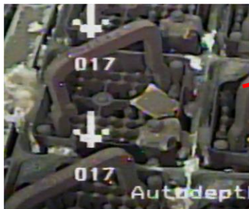
Sandy deposits at the bottom of the cask pit
