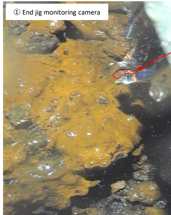
Grasping fuel debris below the opening 2
