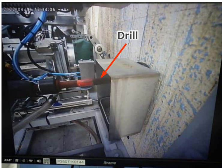
Photo 3. Anchor hole boring
