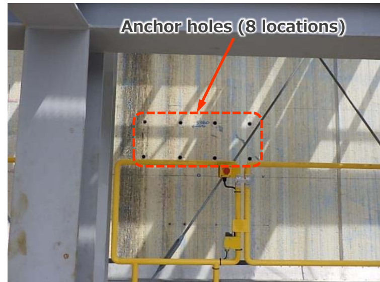
Photo 4. After anchor hole boring
