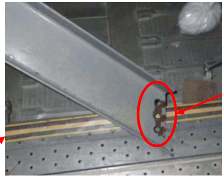
Bolts at the joint ruptured
