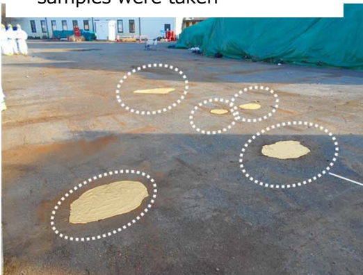
③ Stripper applied to areas where samples were taken
